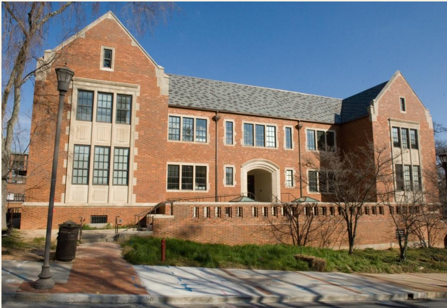
Old Civil Engineering Building Renovation: LEED Gold
