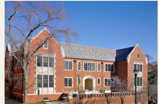
LEED Gold Renovation
